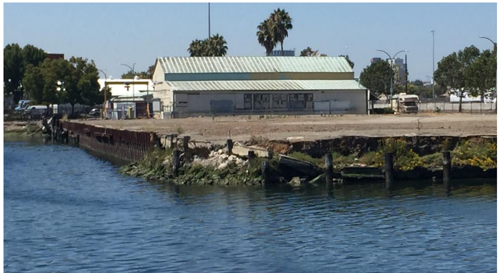
Figure 1. Site Shoreline Conditions
