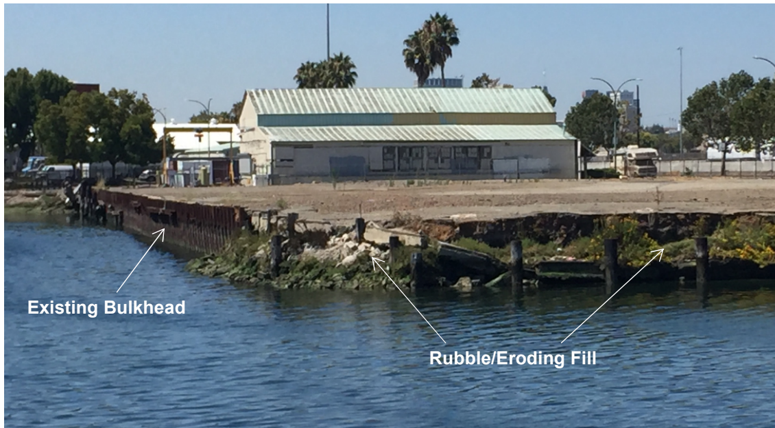
Figure 1. Site Shoreline Conditions
